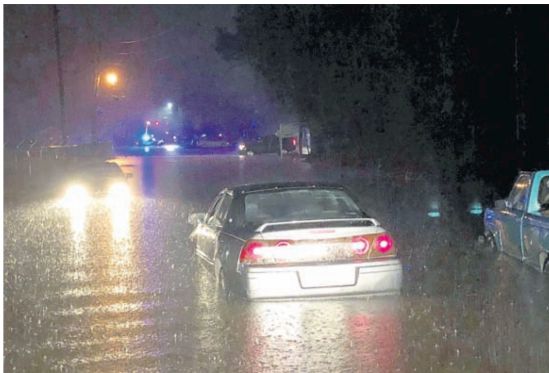
A car fell into this collapsed culvert due to heavy rains on Tommy Butler Road in the Causeyville Whynot area of Lauderdale County, Miss., Friday, Dec 28, 2018.
